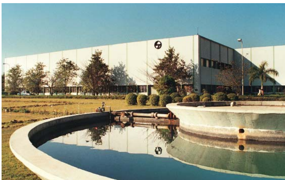
Switchgear Factory, Ahmednagar
