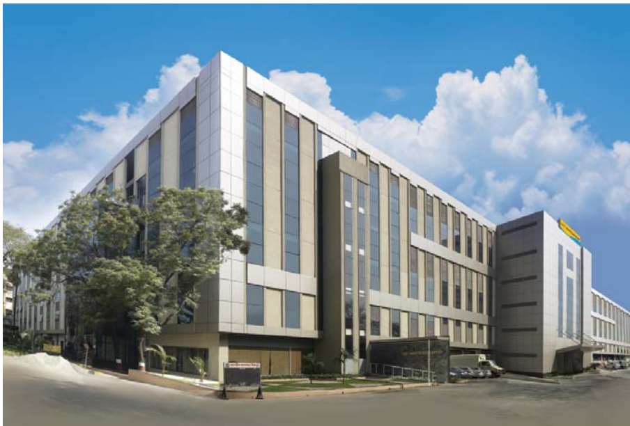
Switchgear Factory, Mumbai
