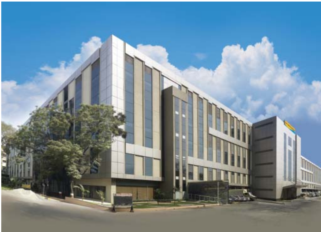
Switchgear Factory, Mumbai
