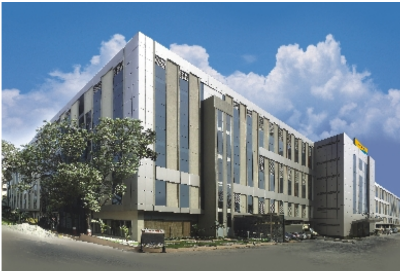
Switchgear Factory, Mumbai
