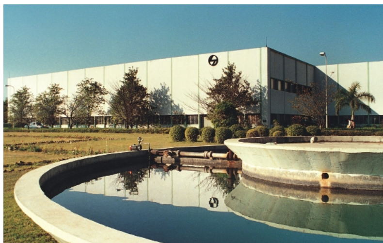
Switchgear Factory, Ahmednagar
